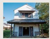
A new storehouse was built early in the Showa Period. It was built above the ground at what appears to be one step higher, possibly as a countermeasure against flooding.
